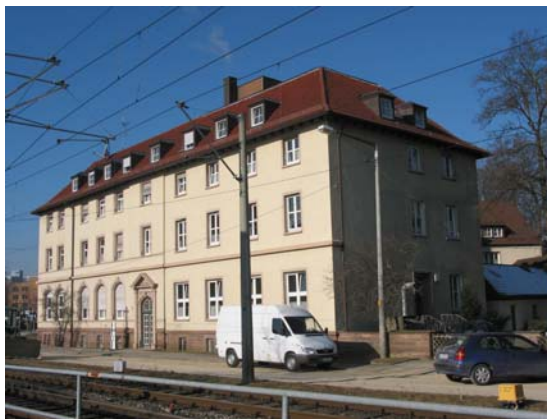
Figure 2: Photo of the German demonstration building nursery home Filderhof in Stuttgart
