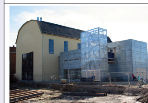
Cultural Centre Proevhallen
